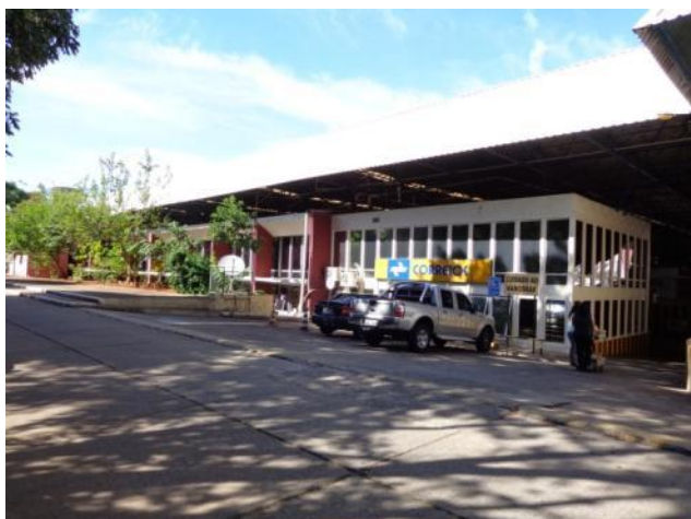
SEEP Bloco 3 (Bloco 09)
