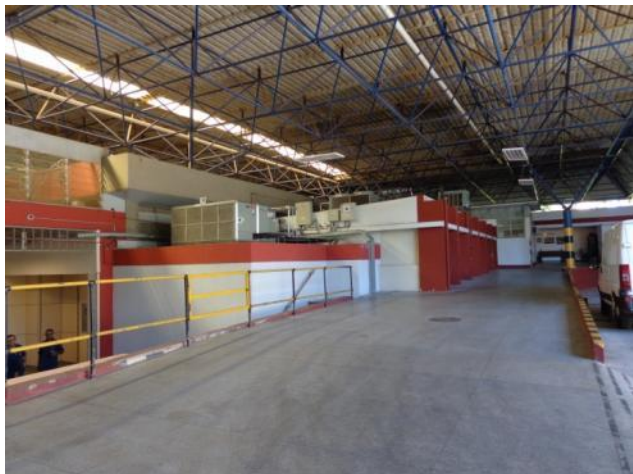
SEEP Bloco 2 e 9 (Bloco 08)
